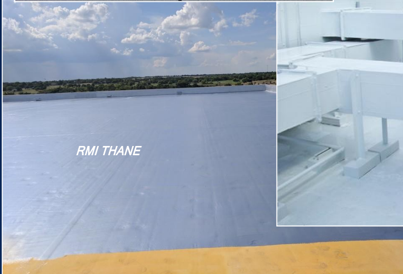
RMI MECHANICAL DUCTWORK RESTORATION
